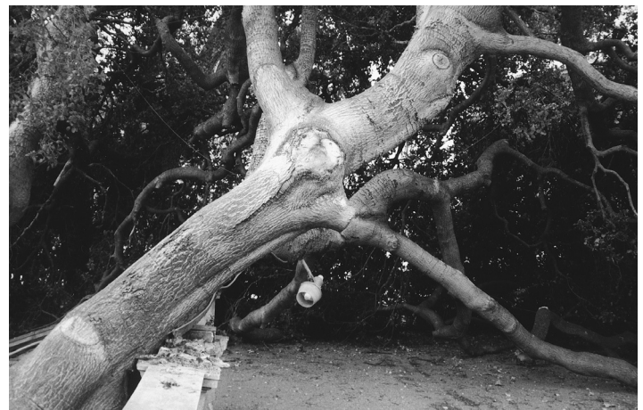
Remnant of the balustrade that was damaged by a falling oak tree in 2001.
